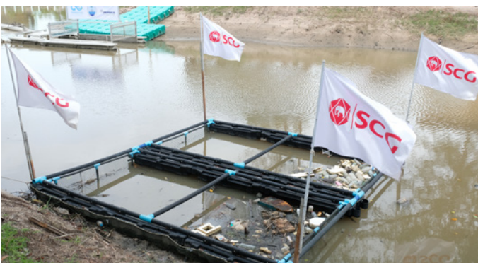
SCG-DMCR Litter Trap Generation 2 using HDPE-Bone
